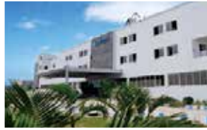
Rudrapur Plant (Green Building)
